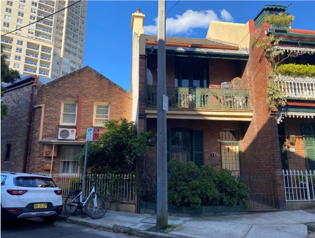
Figure 6. 12 Nimrod Street and adjoining development to the south-east, viewed from south-west
